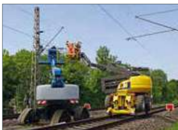
Construction of contact lines
