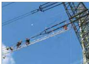
Overhead line construction
