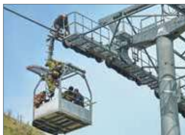
Cable car construction
